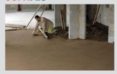
Developed over many years Supaflo\* is at the forefront of screed technology. A flowing screed flooring solution based on a calcium sulfate binder, it provides significant additional benefits such as speed of application, excellent surface finish, accuracy of placement and finishing, reduced thickness and a substantial reduction in movement joints.
