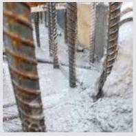
**HOPEFlow Form**<sup>™</sup> is able to flow and consolidate on its own. At the same time it is cohesive enough to fill spaces of almost any size and shape without segregation or bleeding.
