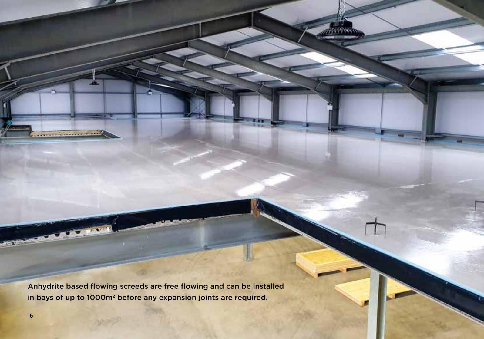
Anhydrite based flowing screeds are free flowing and can be installed in bays of up to 1000m<sup>2</sup> before any expansion joints are required.
